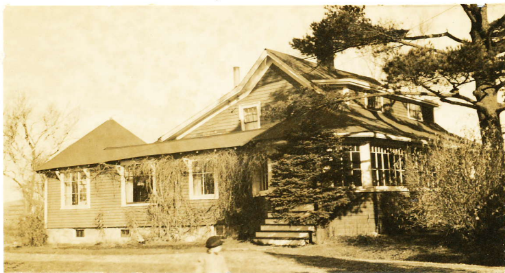
The "Red House", East Riverside, N.B.
