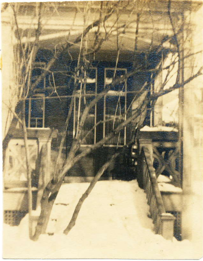
Back verandah, off the Plant Room
